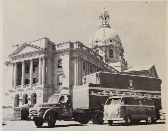
A completely mobile communications system was built by Canadian Electronics for the Alberta Emergency Measures Organization. A large van and one of four satellite vehicles is shown here. The main control van houses telephone and teletype facilities in addition to compact radio equipment linking the four smaller units. The system is capable of forming an effective communications network over any area of disaster.
